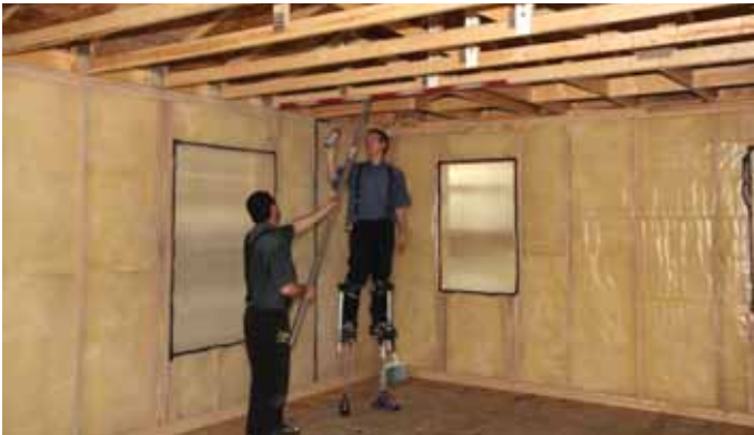
Top: From an observation room, clients can watch the progress of a home under construction in the ProComm's 33,000-square foot production facility. This house measures 71 by 32 feet. The width of the homes is limited by the building's 36-foot wide door. Bottom: Jacoby Kleinsasser and Zach Stahl mark rafters in preparation of the next phase of the home's construction. Opposite page: Completed and nearly completed houses can be seen between the road and the ProComm production facility on the west edge of the Brentwood Colony northwest of Faulkton, S.D.
