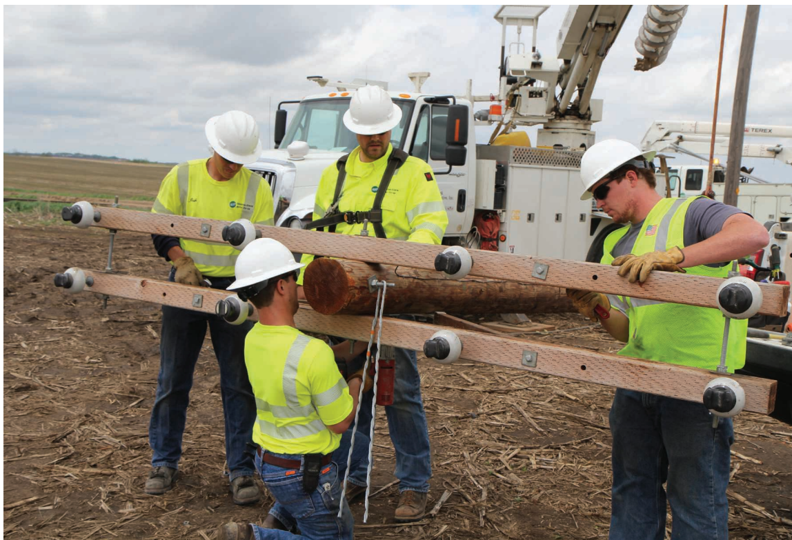
Left: 1,000 hour employee Nick Kramer, right assists a Codington-Clark Electric Cooperative crew with framing a pole for a pole change out south of Watertown in May 2013. Opposite Page: Kramer works on attaching a crossarm as part of the ground work he did during his 1,000 hour experience at Codington-Clark.
