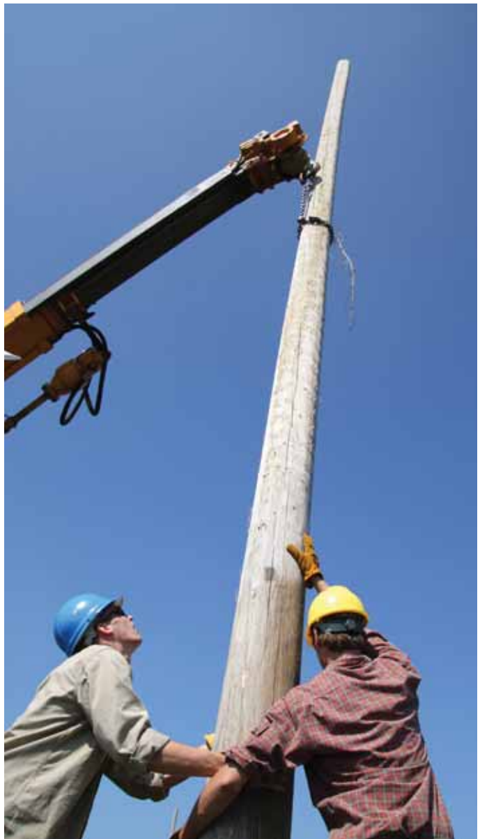
Opposite page: Students practice pole-climbing techniques in Mitchell Technical Institute's Energy Training Center. Above: In MTI's outdoor training field, students practice setting a pole.
